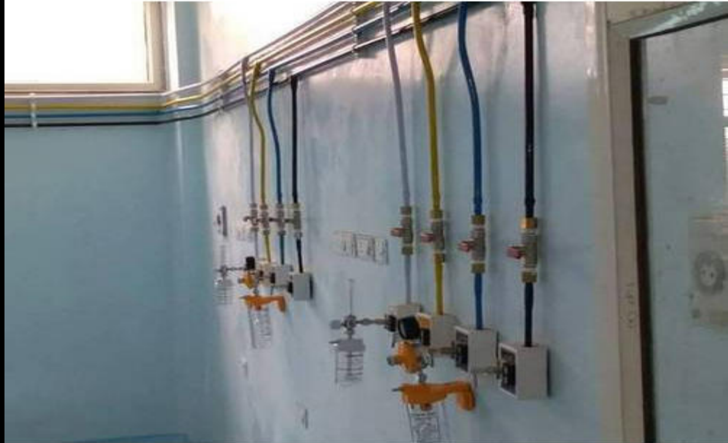
GAS OUTLET SYSTEM IN O.T
